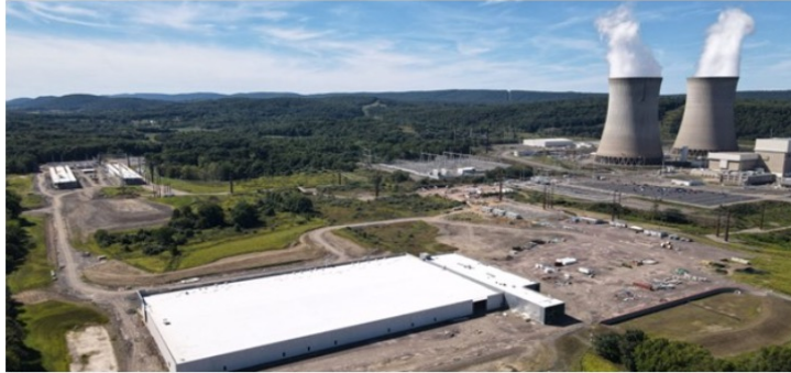
Susquehanna nuclear plant in Salem Township, Penn., along with the data center in foreground. (Photo: Talen Energy)
