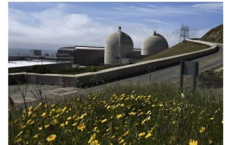
The Diablo Canyon nuclear power plant in Avila Beach, California. Photographer: David Paul Morris
